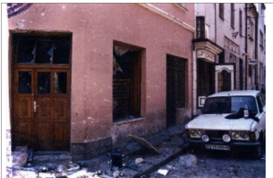
Figure 41 — Facade of the building of cafe Leonardo and the Fiat 125 P after the explosion on 25 May 1995
