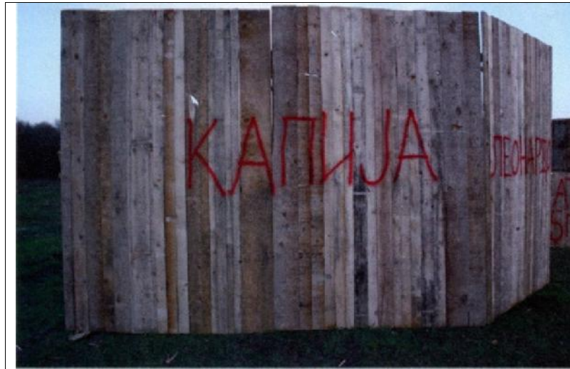
Figure 33 — Screen (wall) of the building of the Kapija STR after the experimental explosion
