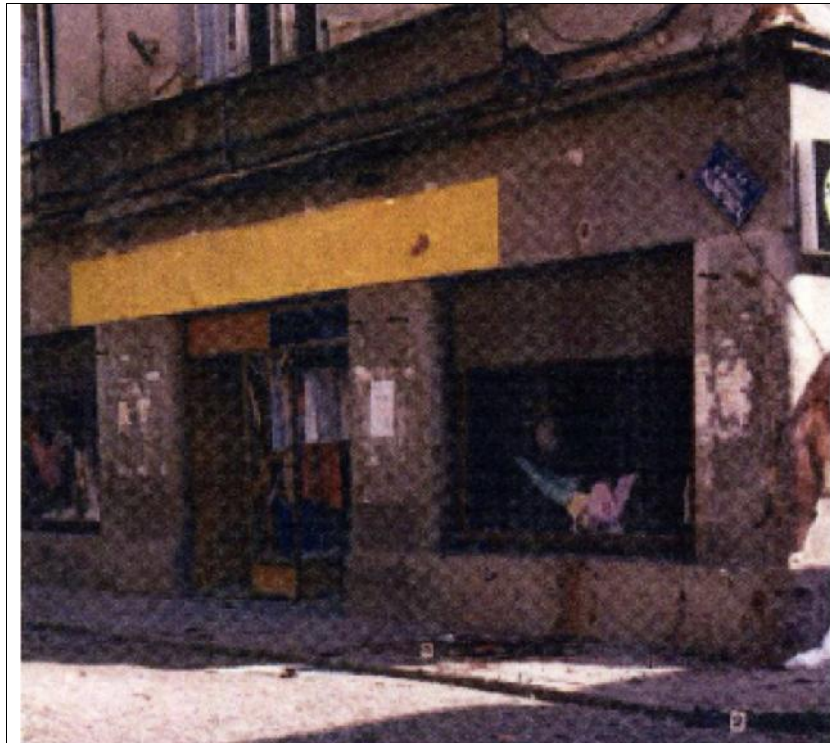
Figure 32 — Buildings on the corner of Mustafe Mu begovi a Street and Partizanska Street after the explosion
