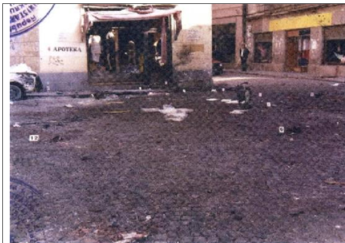
Figure 30 — The building of the NIK shop after the explosion on 25 May 1995
