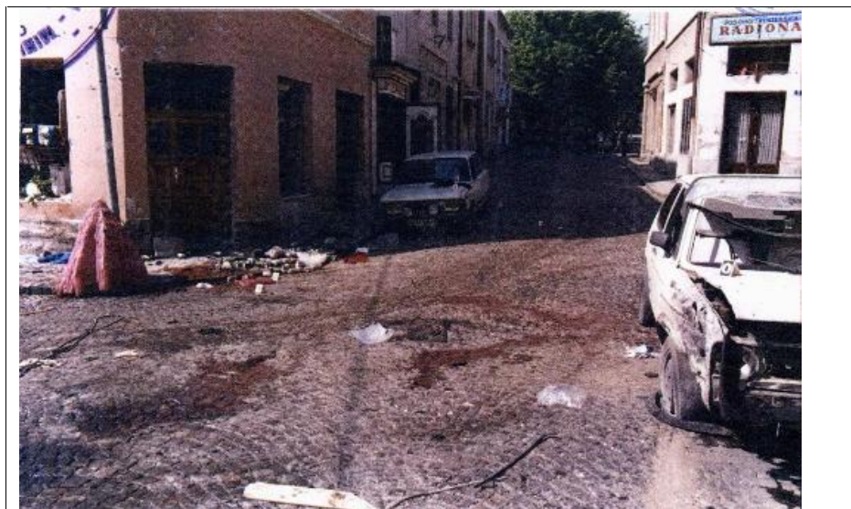
Figure 38 — Corner of the building housing the Kapija STR and cafe Leonardo after the explosion on 25 May 1995
