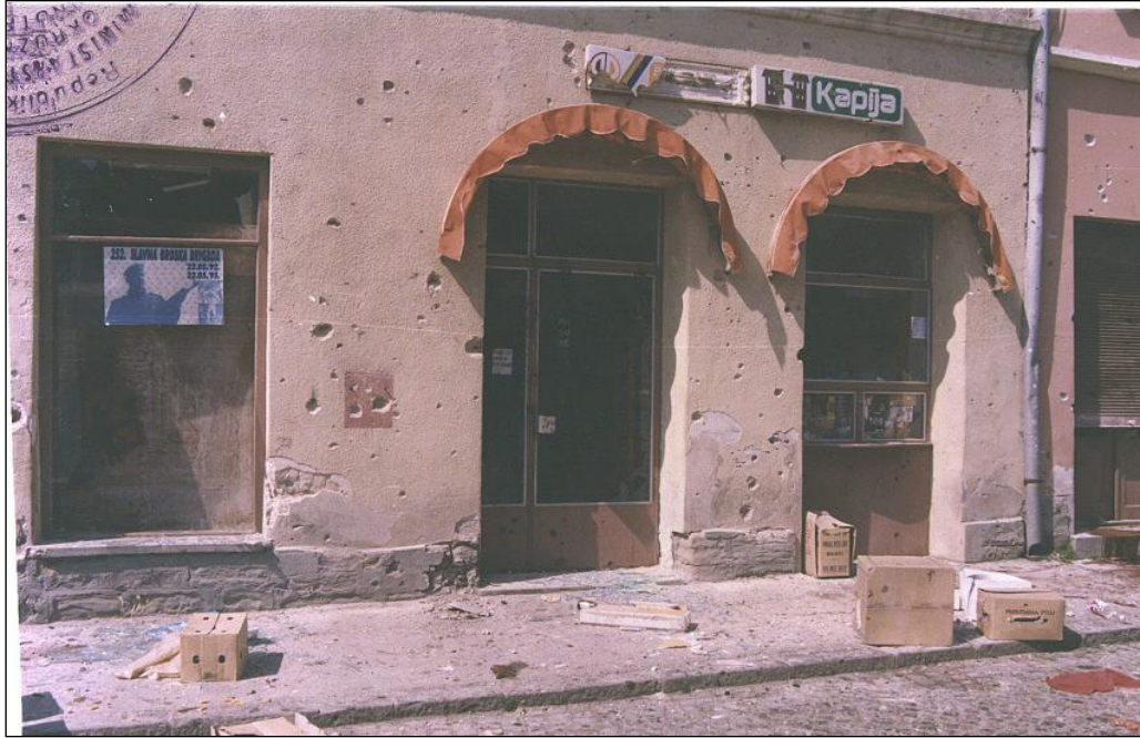
Figure 31 – Appearance of central facade part around "Kapija" premises, on the RCS
