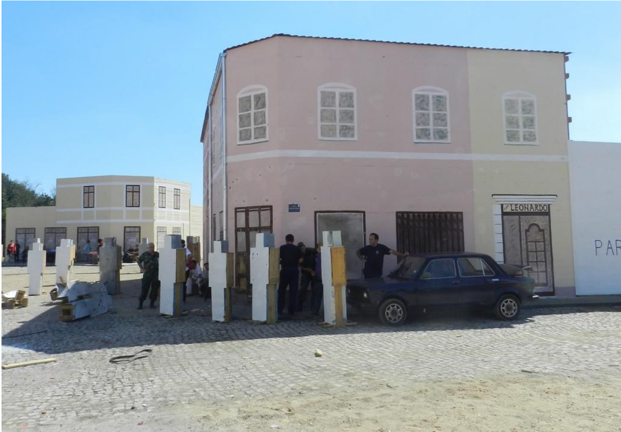
Figure 28 – Appearance of fragmentation action on building corner, left from “Leonardo” cafe, after experimental projectile activation, with visible fragmentation action traces on lower half of building facade, on the corner
