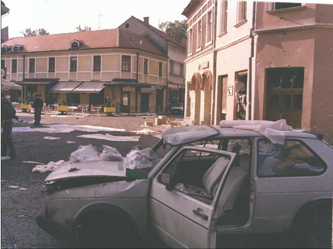
Figure 29 – Fragmentation action appearance on building corner, left from “Leonardo” cafe, on the RCS
