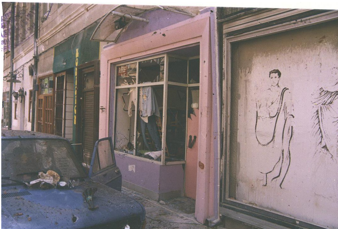
Figure 34 – Closer look on the right part of Partizanska Street, on the place of "Komision" store, with shattered shopwindow, damage to the building facade and parked Z-101 car
