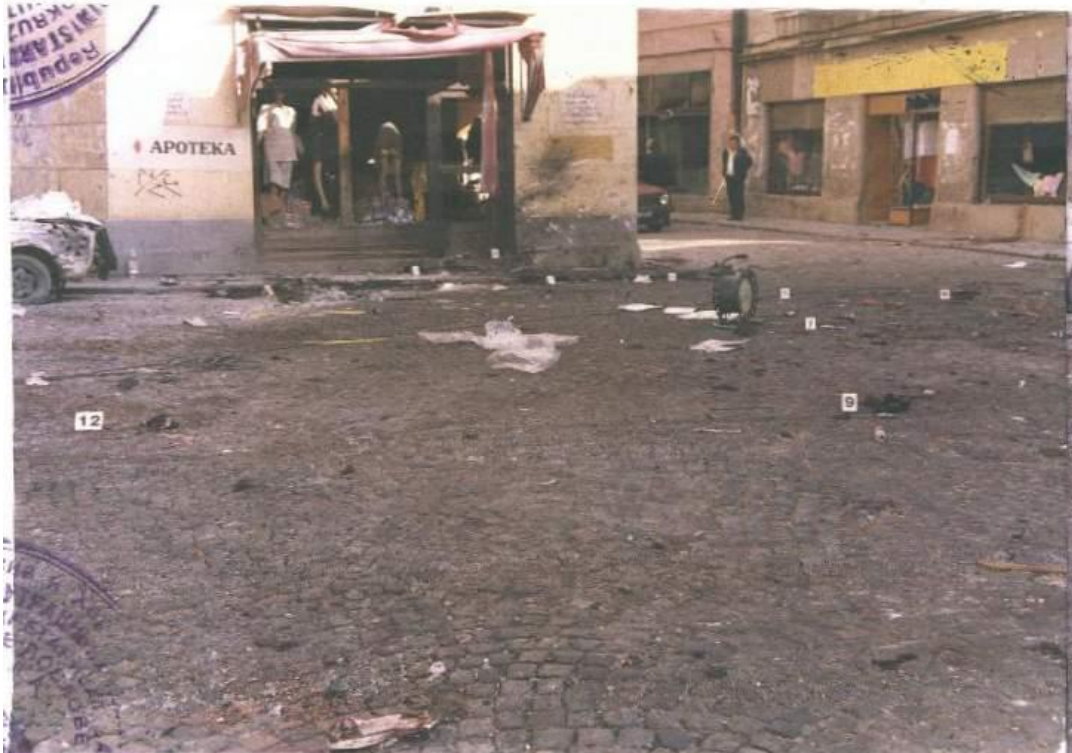
Store window of the actual NIK building after the event, note how the window frame is still in place, and also that the display dummies are still in their upright position
